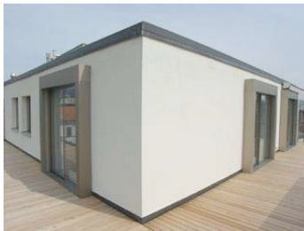
neue Terrasse Attika
